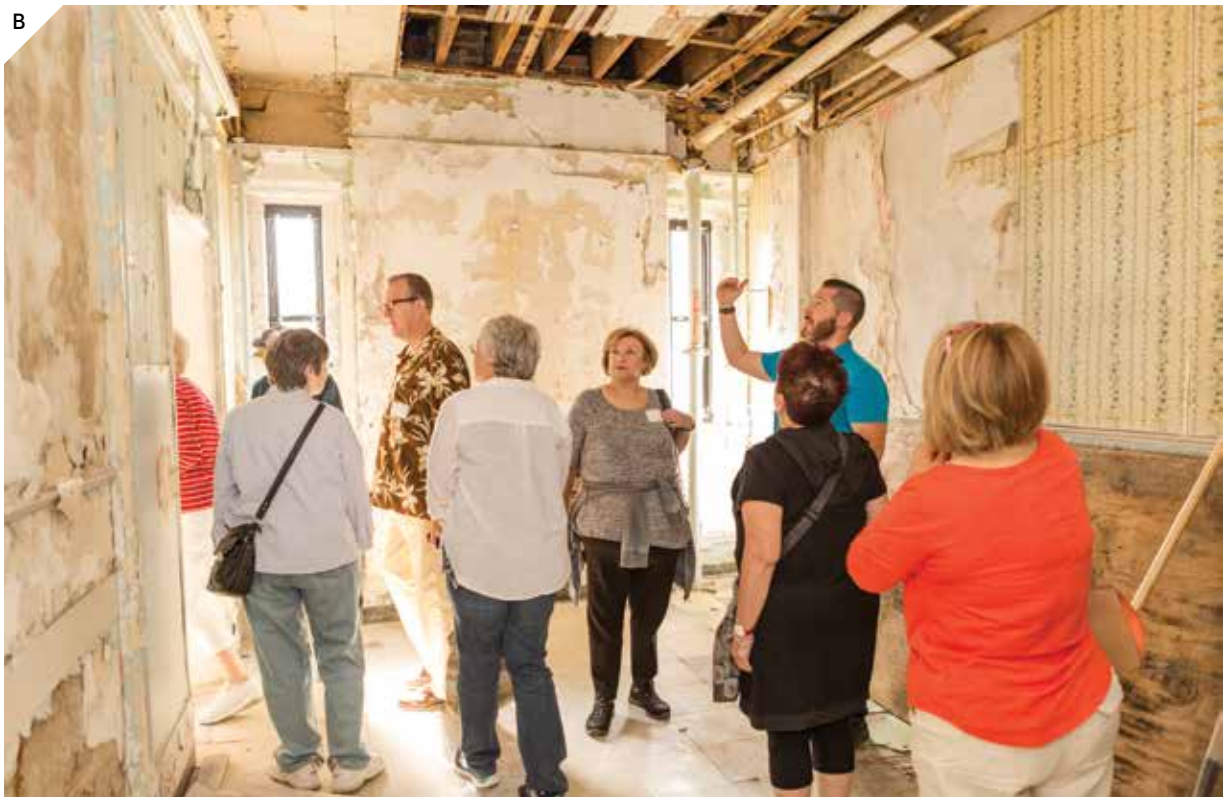
B) Tom Truelson of 1st Choice Roofing leads a group of interested members through the house.
